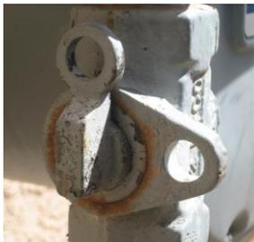
Do not shut off your gas unless you smell gas, hear gas escaping, see a broken gas line or if you suspect a gas leak. Once the gas is shut off at the meter, do not try to turn it back on yourself. If you shut off the gas, there may be a considerable delay before the utility company can turn your service back on. If the gas service shutoff valve
