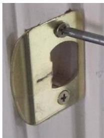
Most strike plates are installed with short screws. When an exterior door is kicked, it can easily be opened because the short screws are an inch deep and are not anchored to the solid 2x4 frame but the decorative trim. An exterior door can be reinforced by replacing the short screws with 3 inch long screws. This will insure the strike plate is properly anchored. If you want to take your home security a step further, purchase a stronger strike plate as well.
