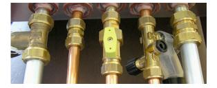
Make sure this valve can be completely shut off. Your valve may be rusted open or it may only partially close. If so, replace it.
